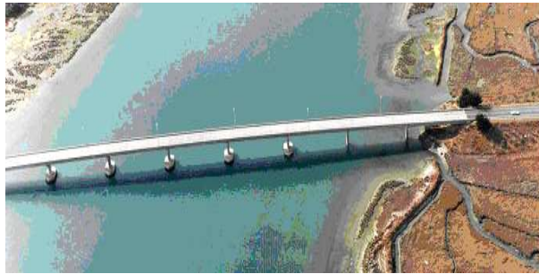
Figure 1. View of Humboldt Bay Middle Channel Bridge (Courtesy of Caltrans)
